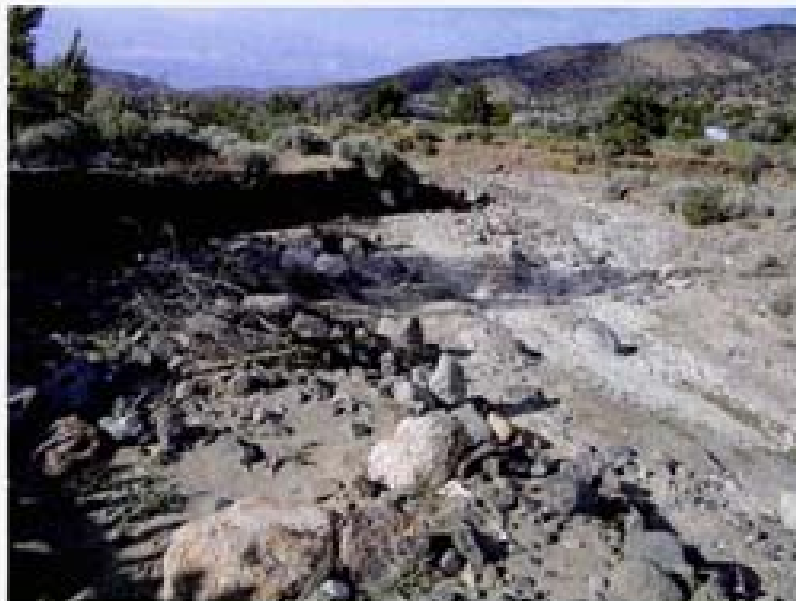
Bank erosion near Moon Lane
